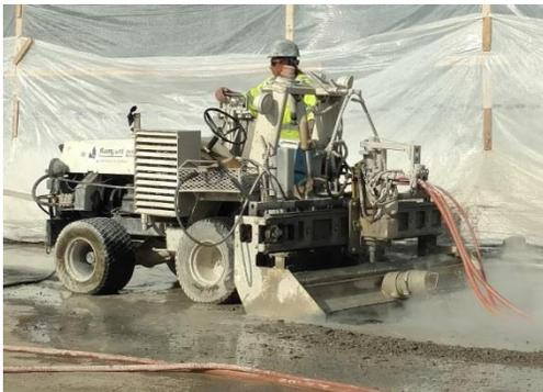
Rampart Hydro Services has been working on a major interstate highway project in Utah. The hydrodemolition work has been happening on I-215 at SR-201 in Salt Lake County. The process is
